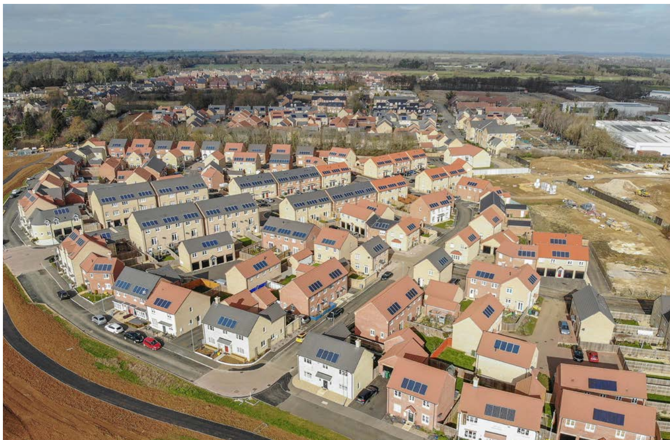
OAKHAM, RUTLAND – multiple phases of commercial and residential built out by the Larkfleet Group 2012 to 2020
